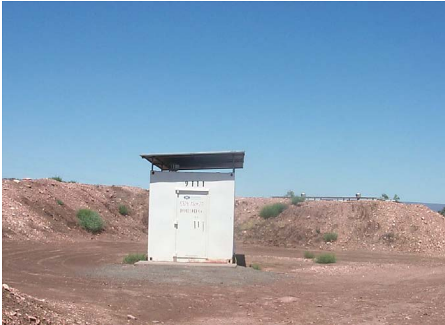
Figure 2: Relocatable magazine protected by earth mounds
