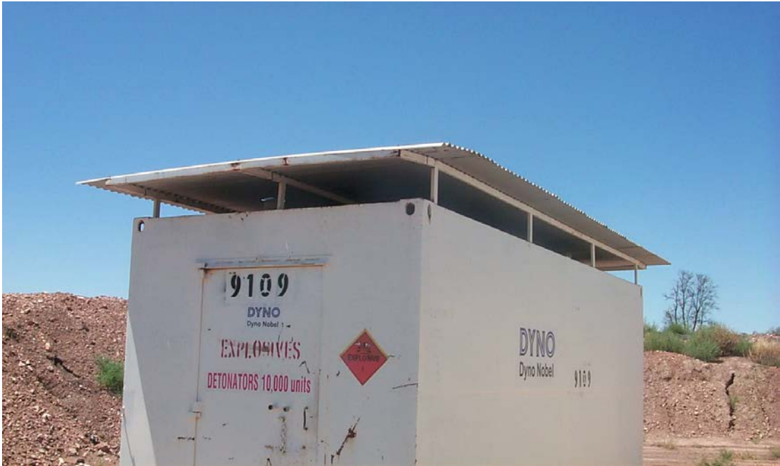
Figure 6: Shade roof on a steel relocatable magazine
